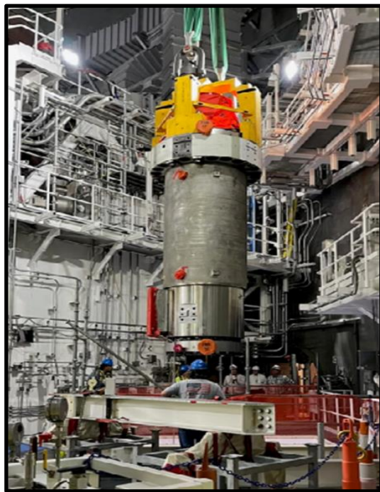
Unit 4 replacement Reactor Coolant Pump
