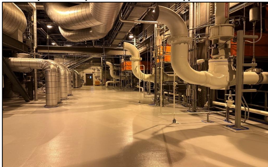
Unit 3 Turbine Building Coating
