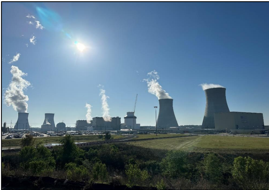
Unit 4 Completed Hot Functional Testing
