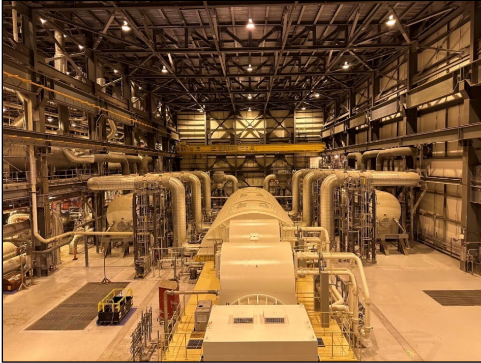
Unit 3 Turbine Building
