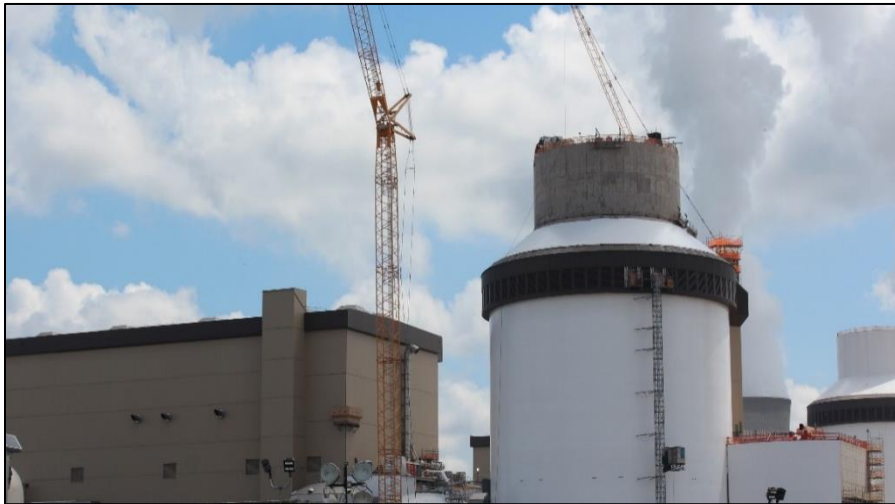
Unit 4 Turbine and Shield Buildings
