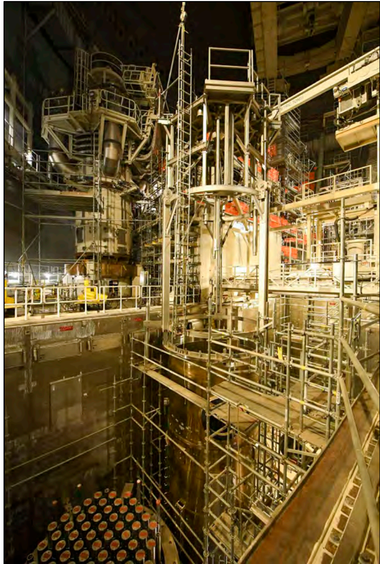
Inside Unit 4 Containment
