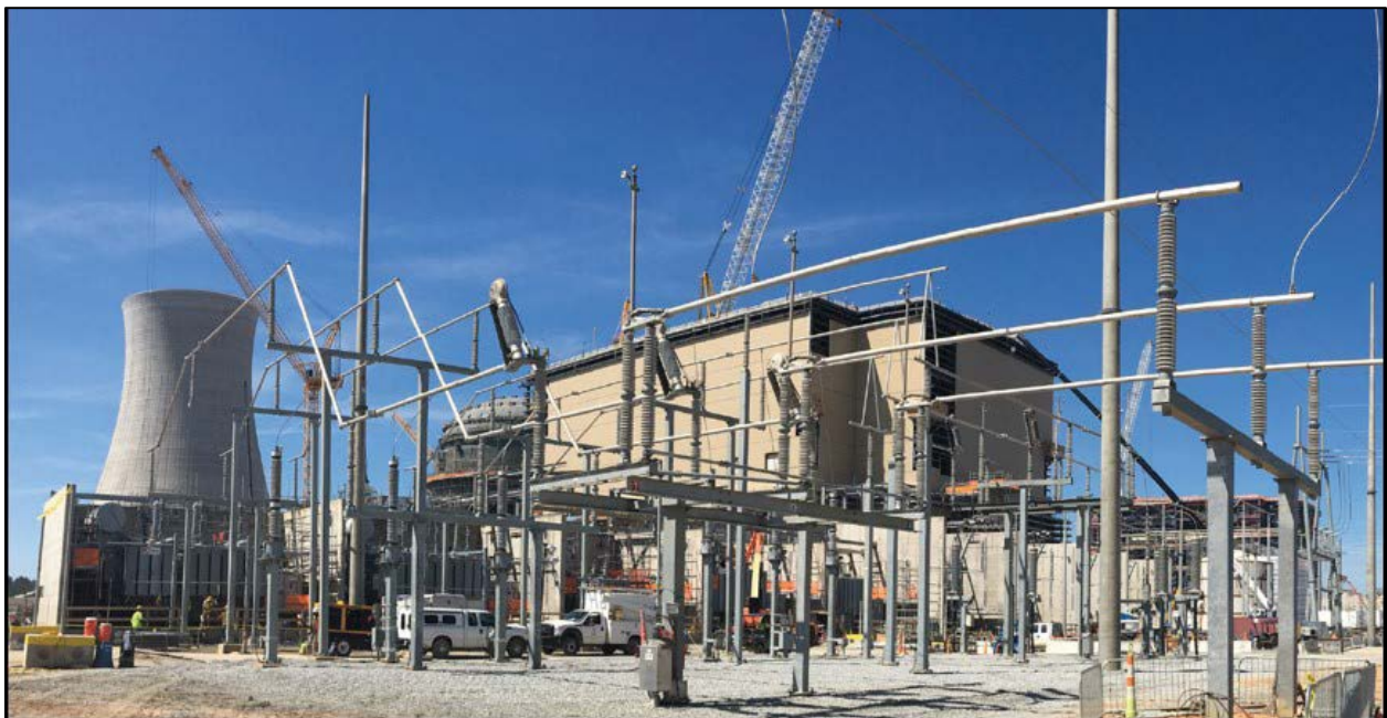
Unit 3 Reserve Auxiliary Transformers for Initial Energization
