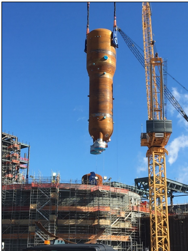
Steam Generator being set inside Unit 4 Containment
