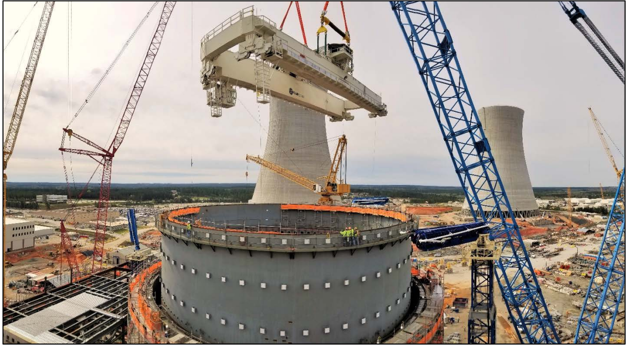
Setting of Polar Crane inside Unit 3 Containment
